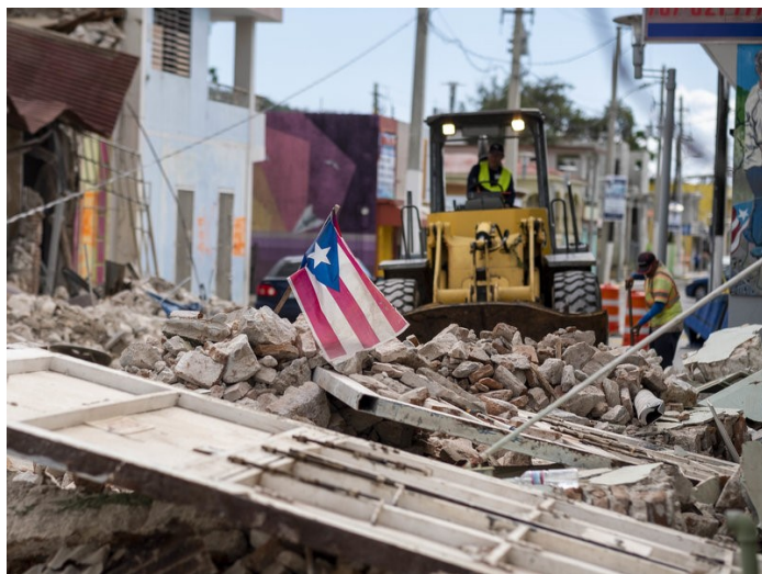
Bull dozer clearing rubble.
